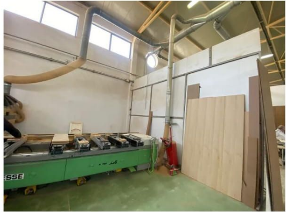
Sistemi i aspirimit te ambientet e brendshme te magazines
