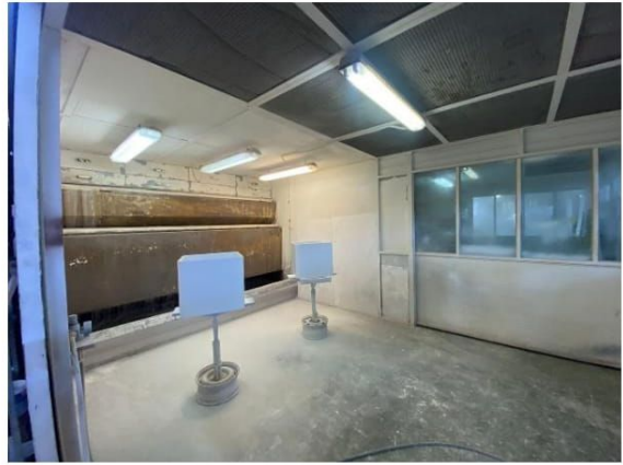
Sistemi i aspirimit te ambientet e brendshme te magazines
