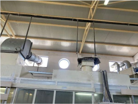
Sistemi i aspirimit te ambientet e brendshme te magazines
